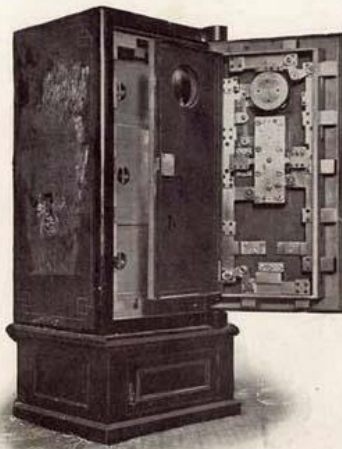
This photograph shows The Chatwood Safe which successfully withstood the severe ordeal recorded on the opposite page. Except for the small hole on the left-hand side, the burglars' attempt proved futile. This is one of the incidents which prove that protection can be given to those who have valuables to protect against every weapon known to science.
